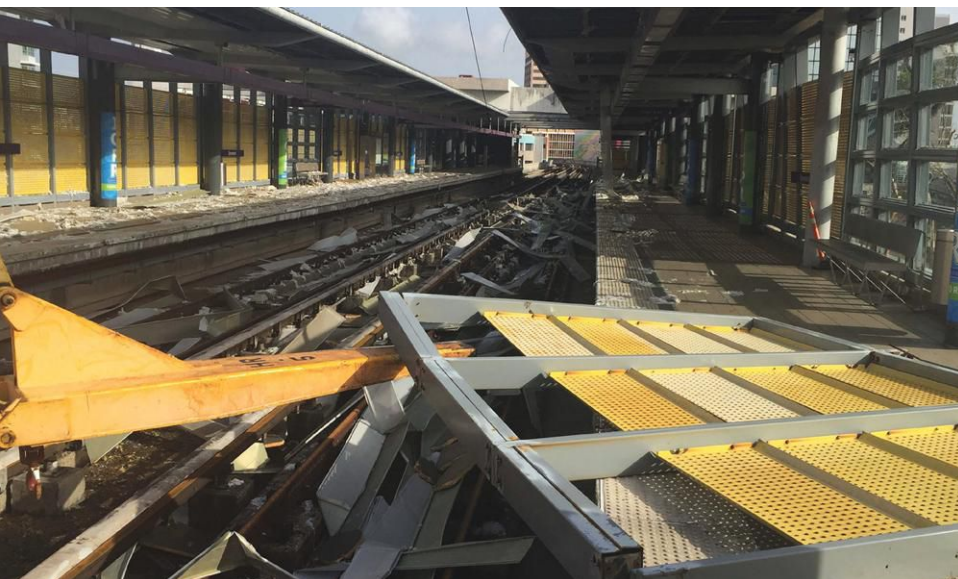
APTIM FEMA PA technical advisors developed robust project worksheets to help the Puerto Rico Dept. of Transportation and Public Works (DTOP) obtain maximum reimbursement for damage sustained to its assets.
