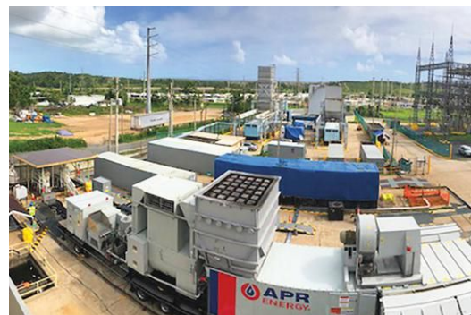
The APTIM team provided 25 MW of time-critical generator power to support electricity restoration in Puerto Rico after Hurricane Maria.
