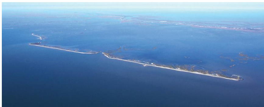
Innovative procurement and management strategies enabled the firm to construct 15 miles of emergency sand barrier berm in eight months to protect coastal Louisiana from the Deepwater Horizon oil spill.
