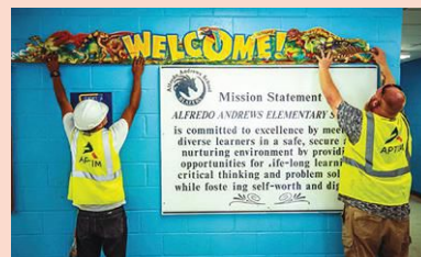
APTIM performed temporary repairs and cleanup of schools in the U.S. Virgin Islands impacted by hurricanes Irma and Maria.
